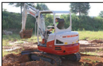
construction full acier
